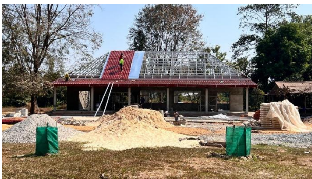
Construction of the Main Hall
