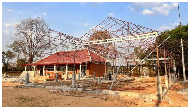
Reconstructing the former Greenhouse to become an Open Hall
