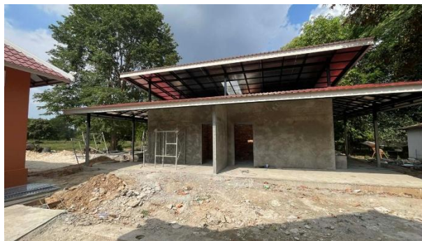
Construction of Toilet and Bath Building
